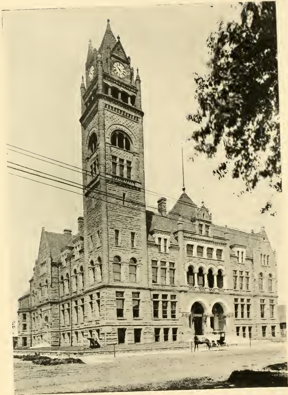
CITY HALL AND PUBLIC LIBRARY, BAY CITY, E. S.
